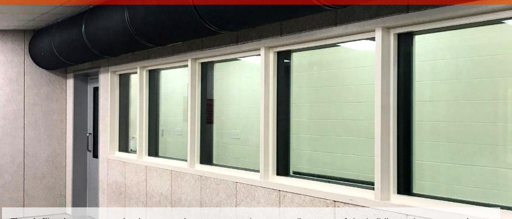
The air filtration system maintains a negative pressure to the surrounding areas of the building to keep contaminants from entering the control area. The average air flow is 75 cubic feet per minute with no readings less than 50 cubic feet per minute. The area is maintained to a negative condition of .05" of static pressure.
